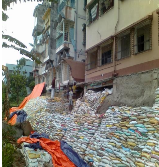
Figure:1 - Sand filled bag dumping
