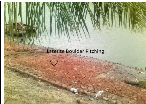
Figure:6- Laterite Boulder Pitching
