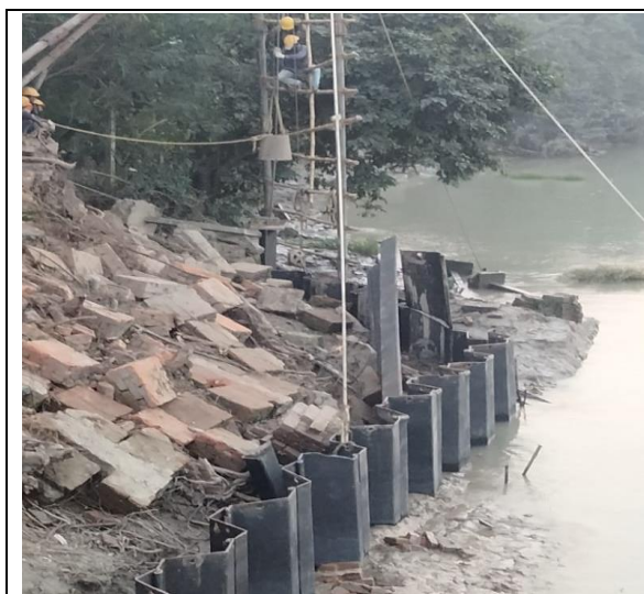
Figure:13- Sheet Pile Wall
