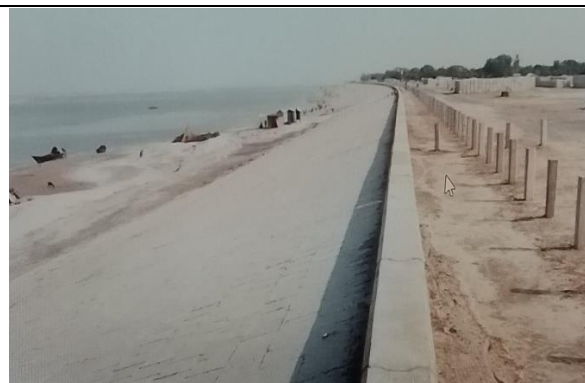
Figure:6- Laterite Boulder Pitching
