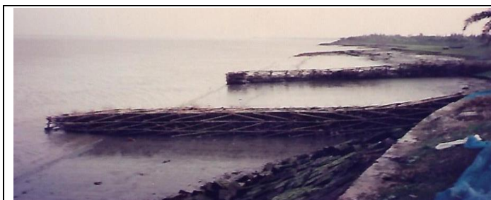
Figure:5 – Semipermeable Spurs
