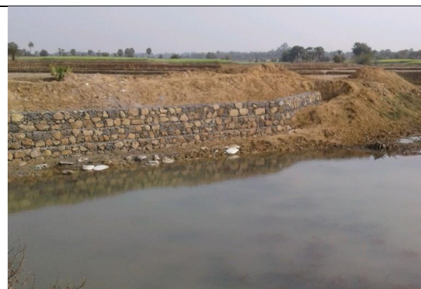
Figure:11- Gabion wall
