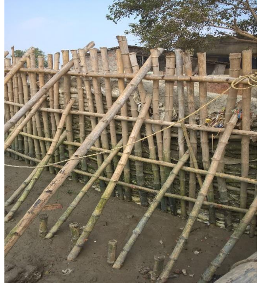
Figure:2 – Bamboo piling
