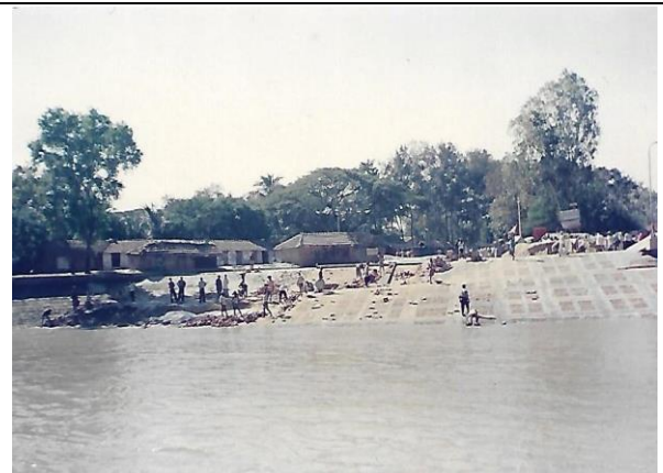
Figure:7- Brick Block Pitching
